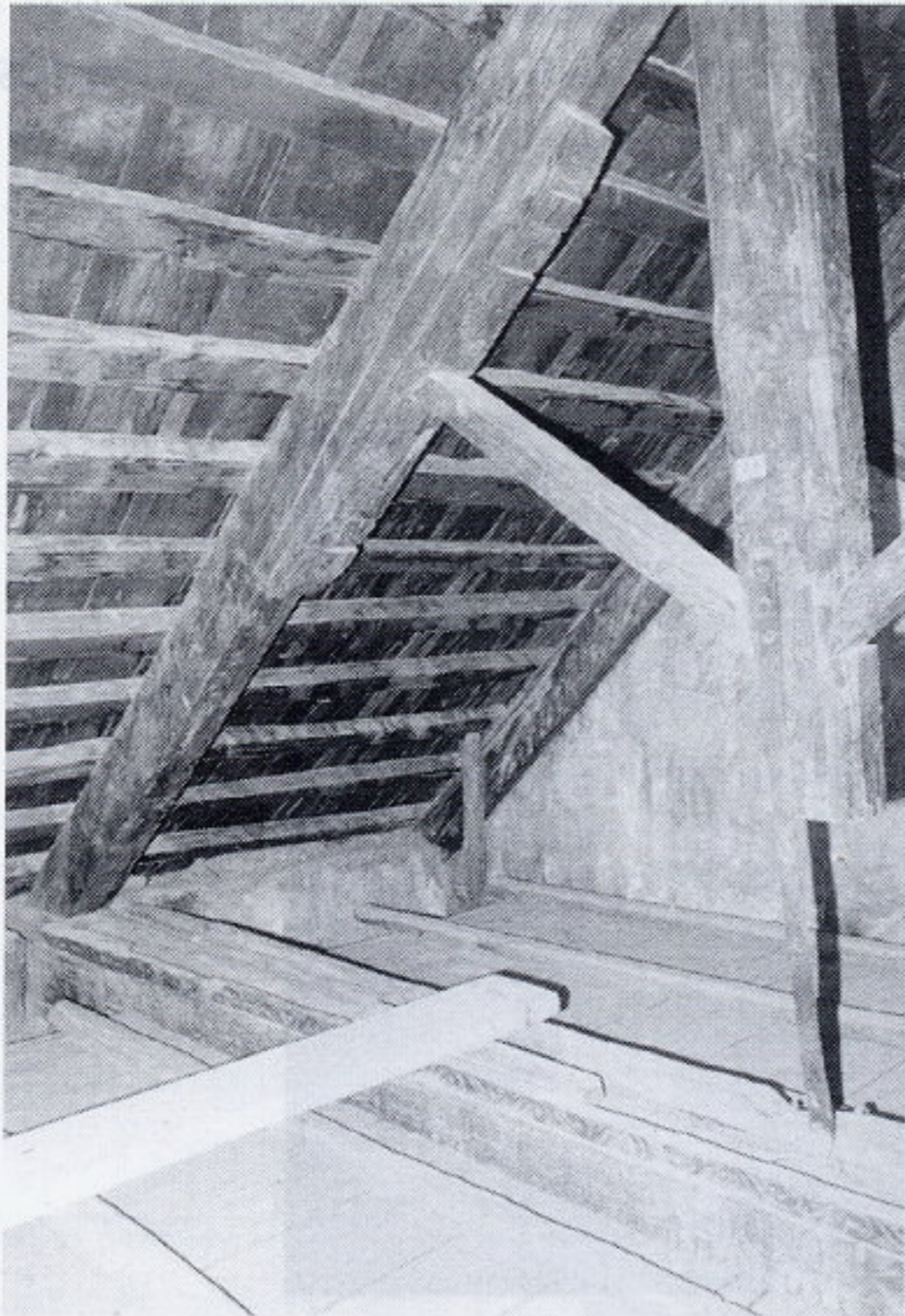
Figs. 4 and 5. Views of the interior of the roof of the central nave showing original trusses no. 2 and no. 9, purlins, decking and the ridge beam.
