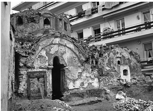
Fig. 2. View from S (1973).
