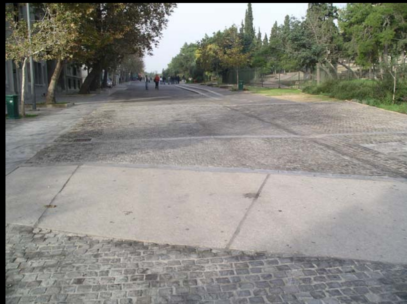
Dionysiou Areopagitou St. pedestrian precinct: Materials used for the construction
